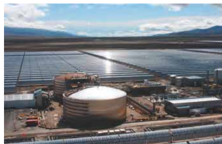
Andasol 1: 500 000 square metres of mirror surface capture the sunlight ©Solar Millennium AG
